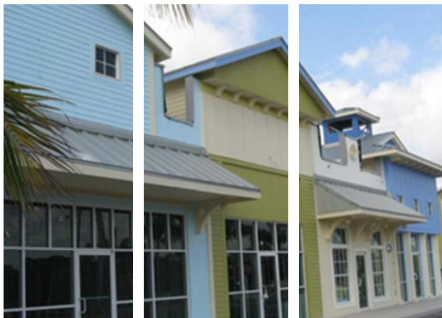
Figure 4.3.3: The use of windows, roofs and roof lines, colors, and material changes using Florida Vernacular.
