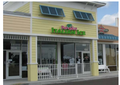
Figure 4.5.2: Florida Vernacular “Commercial” porch / colonnade.
