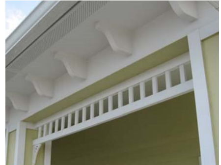
Figure 4.5.1: Gingerbread trim and/or porch railings, columns or posts must be constructed of wood, aluminum or rustproof metals, composite materials, or other traditionally accepted Florida Vernacular materials to create the appearance of light framed wood construction
