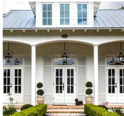
Figure 1.2.2: Example of “Traditional” Florida Vernacular Architecture.
