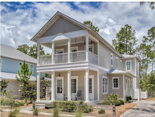
Figure 1.2.1: Example of “Traditional” Florida Vernacular Architecture.
