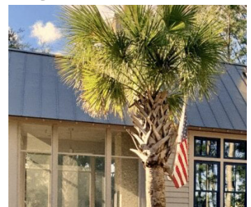
Figure 4.4.3: Example of Florida Vernacular Style “mansard” roof.
